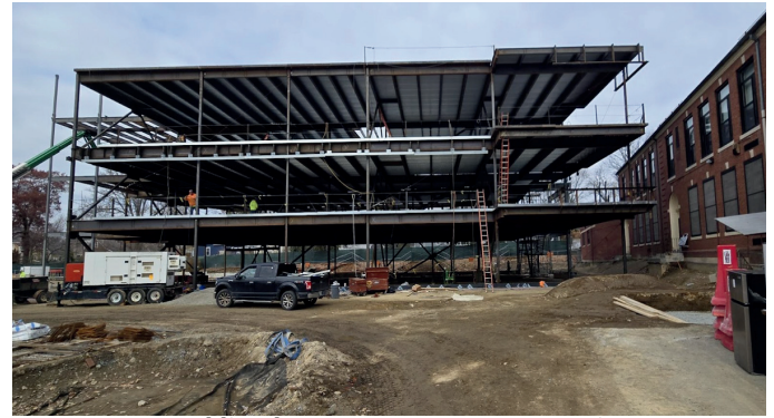
Franklin Elementary New Construction
