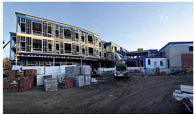
Countryside Elementary New Construction
